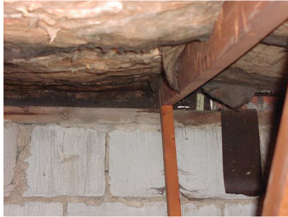
Figure 1: Truss leaning
